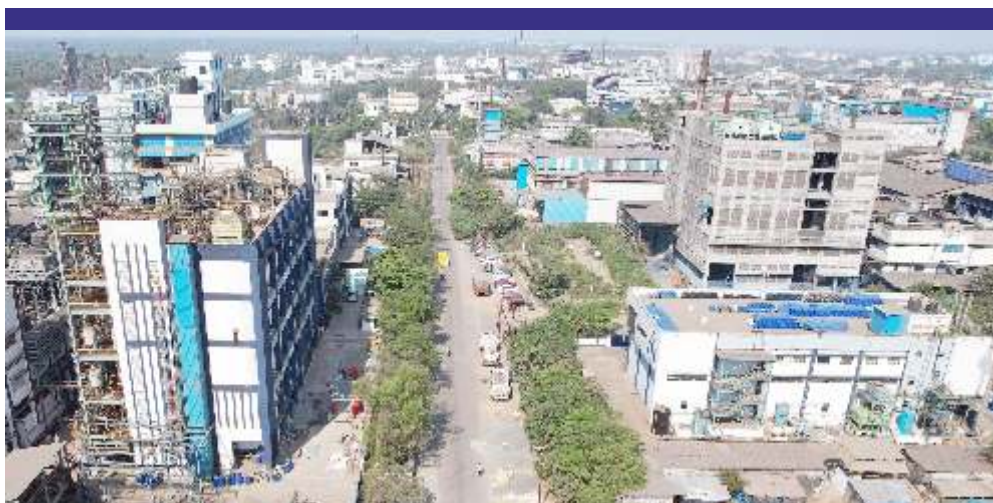
VUE DU CIEL SAREX OVERSEAS MANUFACTURING COMPLEX, TARAPUR, INDIA
