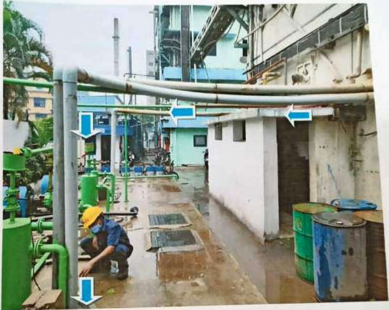
Piping From Quality Control Building And Drying Packing Building To Under Ground Water Storage Tank
